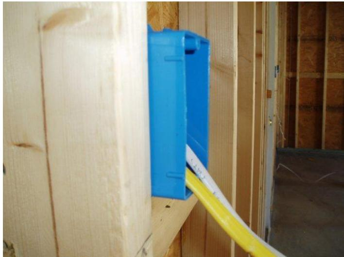
**Cutting for electrical boxes.** This is probably the most challenging part of a slatwall installation. The most important rule is “measure twice, cut once” because you typically do not get a second chance to get the hole in the right place.
