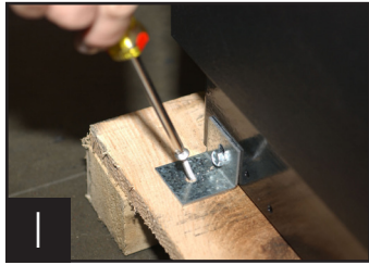
Removing bracket from skid.
