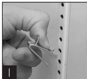
Installing top tab of shelf clip
