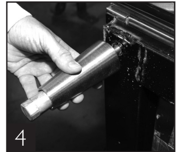
4 Thread leg into cabinet bottom frame rail.
