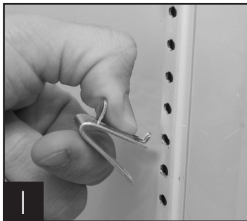
1 Installing top tab of shelf clip
