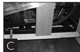
Removing skid from bottom of cabinet.
